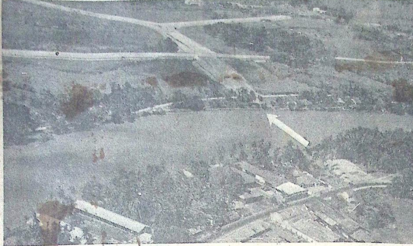
Site of New Kelani Bridge 21/12/51
